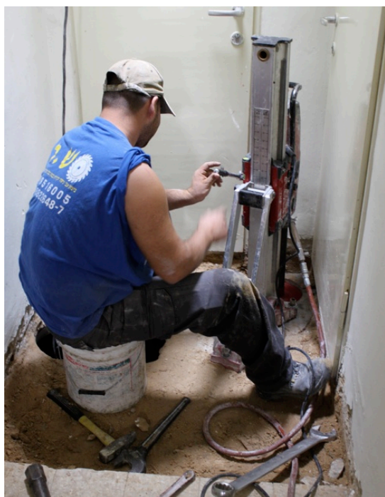
Figure 11. Drilling probe holes into the tomb
