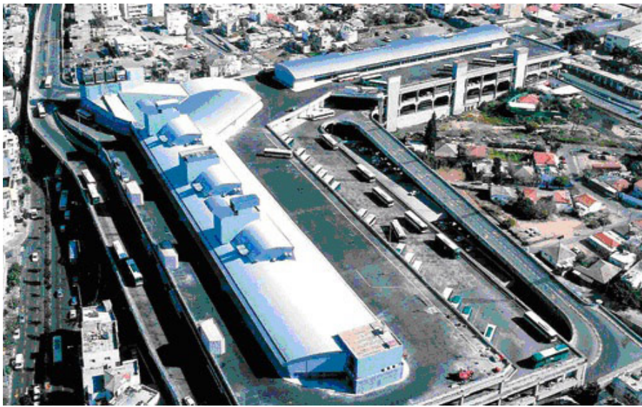
Figure 46: General View of the Tel Aviv Central Bus Station
