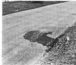
.b. Medium-severity patching
