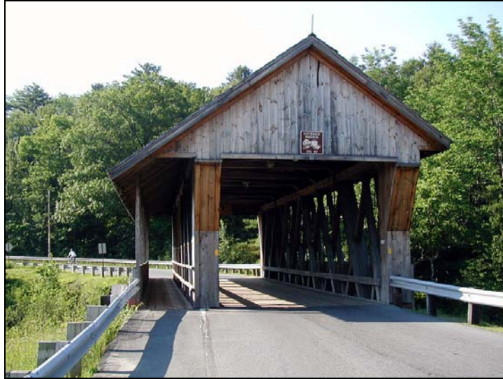
Covered Bridge with separated path. www.pedbikeimages.org/ Dan Burden, 2006
