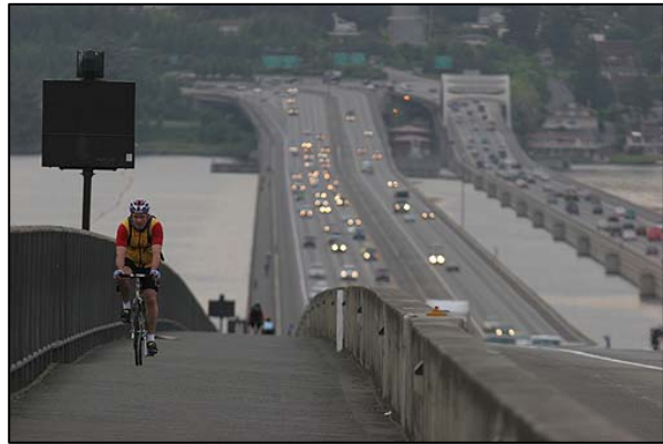
I-90 floating bridge across Lake Washington in Seattle
