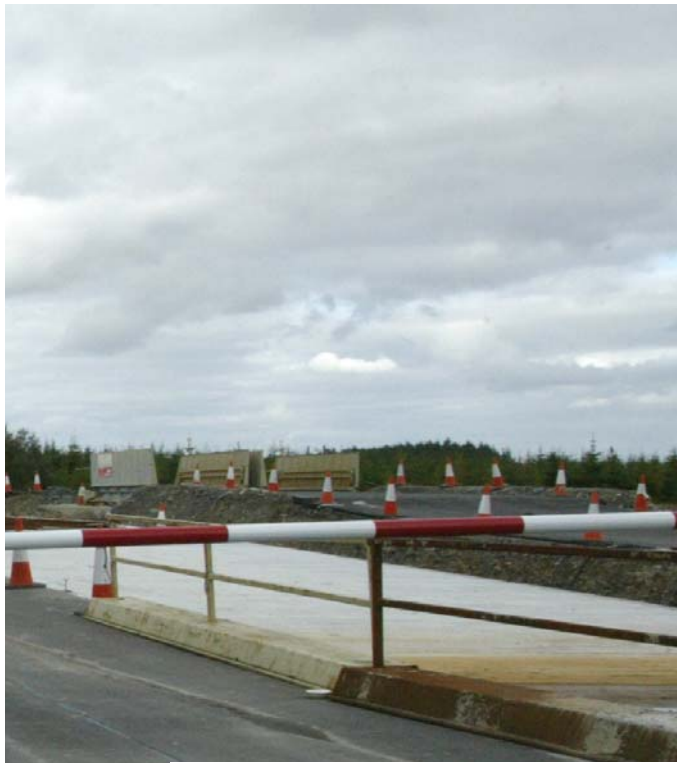
Entrance to the proposed processing plant at Ballinaboy
