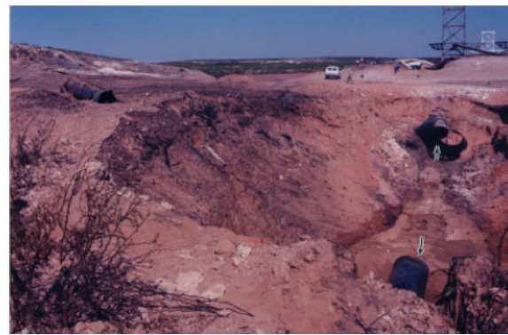
FIGURE 11. CARLSBAD RUPTURE CRATER (COURTESY OF NTSB)
