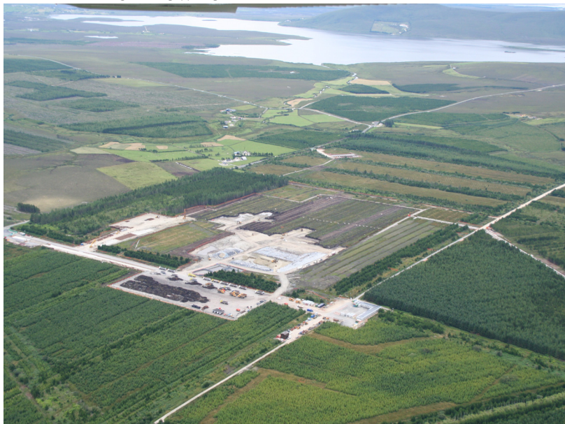
FIGURE 19. GAS PLANT SITE LOOKING TOWARD CARROWMORE LAKE
