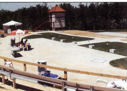
Exterior views of three of the permanent projects in which ACOG invested are shown above. top: Olympic Stadium center Stone Mountain Park Tennis Center bottom: Wolf Creek Shooting Complex
