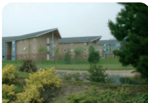
Completed SLAM accommodation at RM Poole
