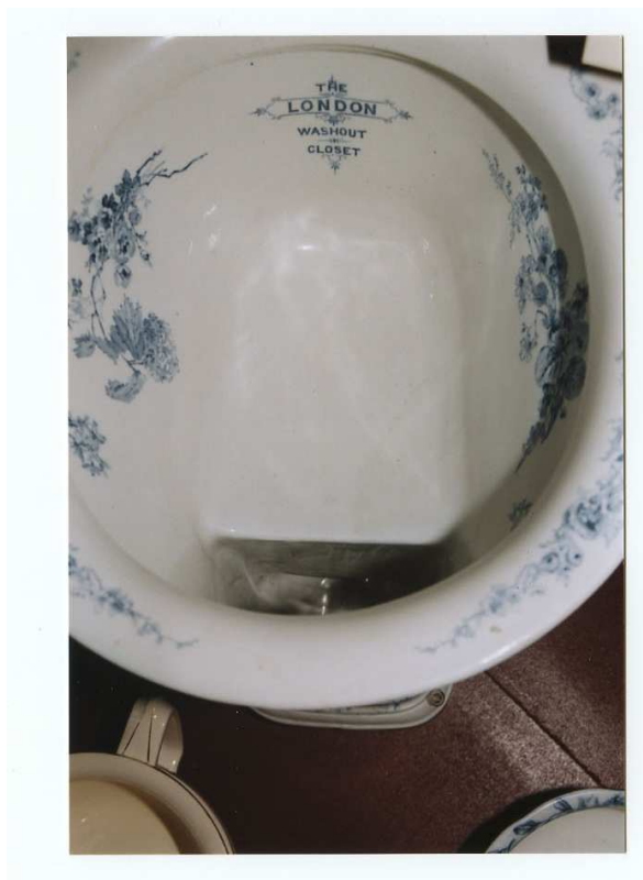
Figure 10 Wash-out Closet
