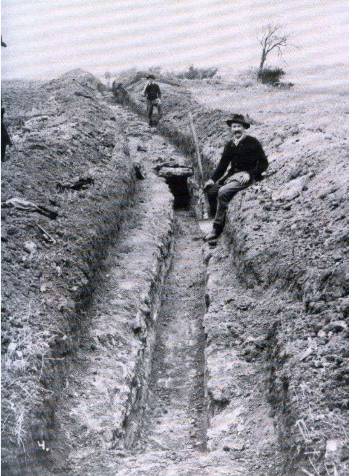
Figure 26 Trenches for the laying of sewerage pipes
