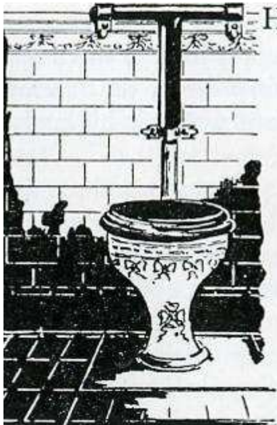
Figure 44 The first W.C. (1592) which included a cistern
