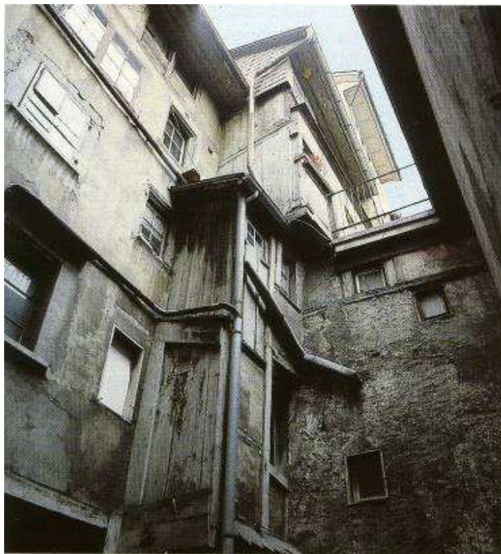
Figure 24 Garderobe with soil and rainwater pipes
