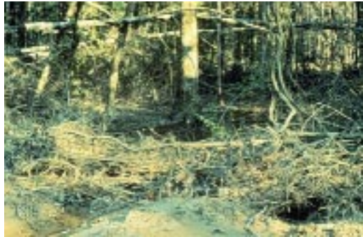
Figure 12. Debris deposited in stream channel
