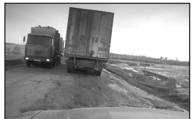
The weak link in Russia's largest highway: patches of missing asphalt slow traffic to a crawl for a few hours outside of Novgorod.
