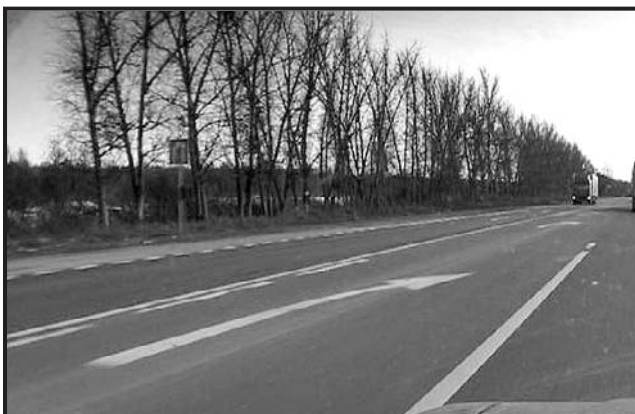
A sign of hope? This section of the Moscow - St. Petersburg highway finally gets a passing lane and fresh coat of paint.
