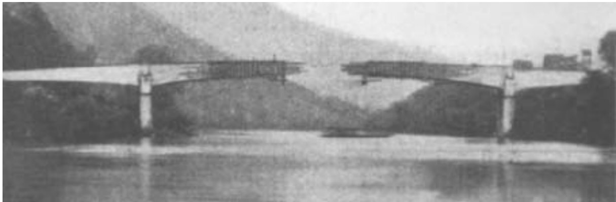
Fig. 42: First reinforced concrete bridge built using the cantilever construction method over the Rio de Peixe in Brazil, Emilio Baumgart, 1930. (Deinhard)
