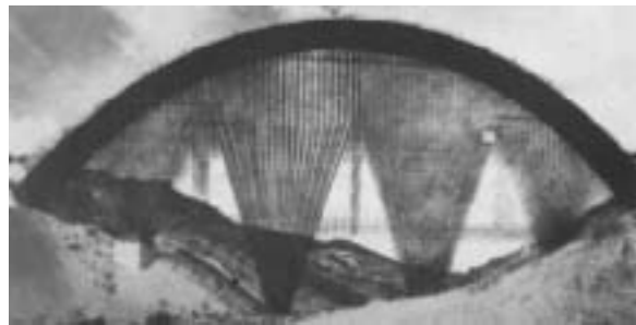
Fig. 35: Centering for the Aglio Viaduct for the motorway between Milan and Naples, Italy. 164 m span, 44 meters high. (Wittfoht)
