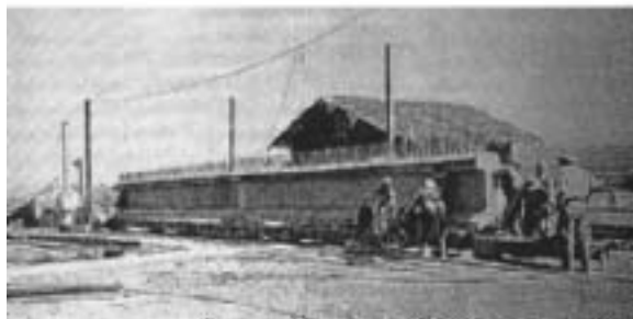
Fig. 21: Prefabricated prestressed I-girder bridges for a service footway on the weir of the Wadi Fodda River, Freyssinet, 1937-1939. (a) General section of weir and footbridge. (b) Pre-cast girder before installation showing ends of the stirrups that will monolithically connect the deck slab to the girder. (Grote and Marrey)
