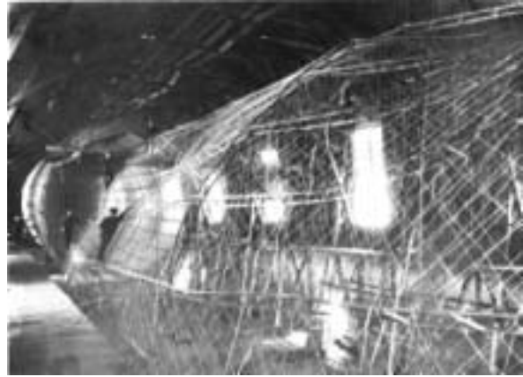
Fig. 23: View of damage done to LZ-1 when an apparatus in its shed broke. (Knäusel)
