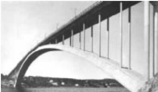
Fig. 6: The Sandö Bridge over the Ängermändälv, Sweden with a 269 m span, Skanska Cementgjuteriet AB, 1942. (Wittfoht)
