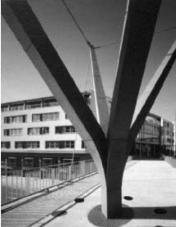
Fig. 25: Stone mast of a cable supported pedestrian bridge in Bad Homburg, Germany. Schlaich Bergemann & Partner, 2002. (Russell)
