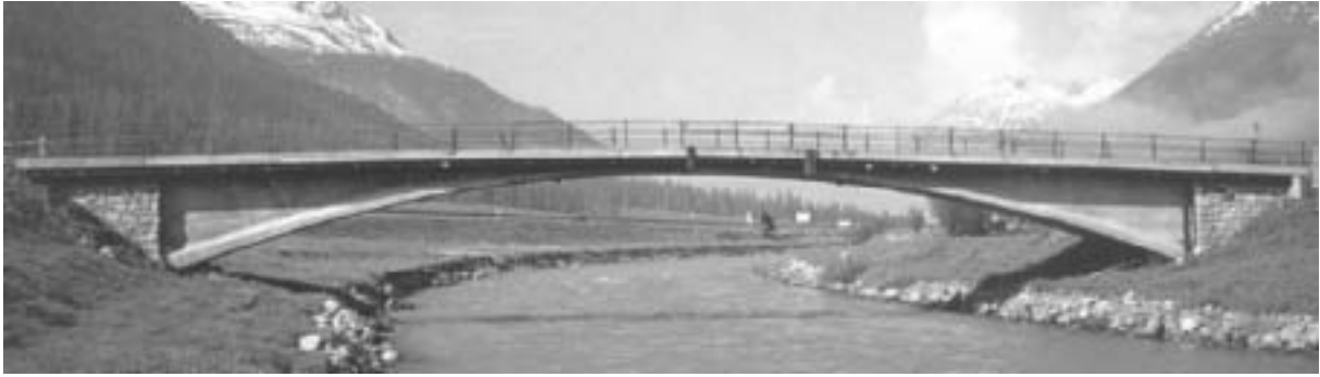
Fig. 36: Zuoz Bridge, first reinforced concrete box section bridge with plain spandrels, Robert Maillart, 1901. (Brown)
