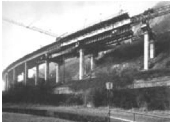
Fig. 49: Krahenberg Bridge, first prestressed concrete bridge built using span-by-span cantilever construction method with self-supporting traveling formwork. (Wittfoht)
