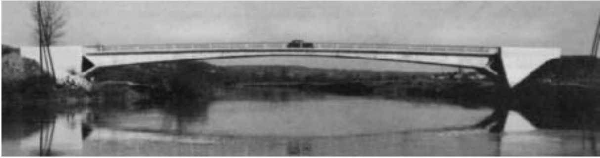
Fig. 28: Marne Bridge at Ussy, Freyssinet. (Wittfoht)
