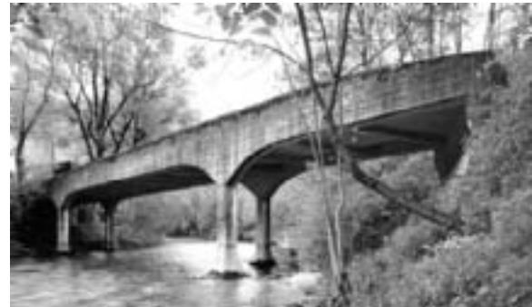
Fig. 15: Liesberg Bridge, three-span continuous reinforced-concrete beam bridge, Maillart, 1935. (Billington)
