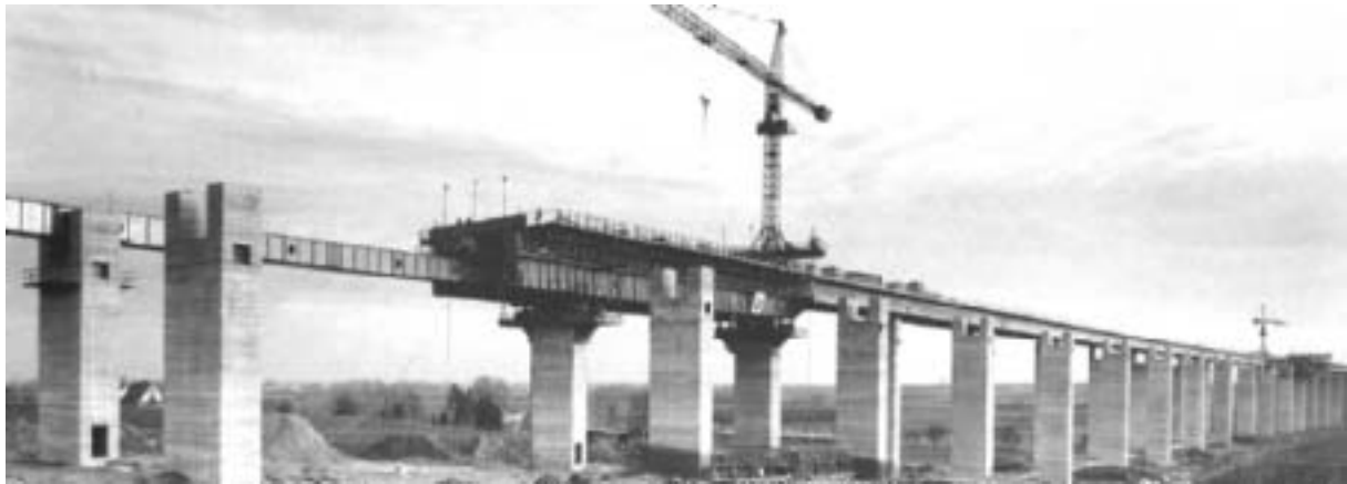
Fig. 46: Example of traveling girders that support formwork from below the bridge deck. Note the openings provided for at the top of the piers to allow the traveling girder to pass. Image shows the construction of the 1.5 km Pfeddersheim Viaduct for the A 61 between Ludwigshafen and Krefeld, Germany. (Wittfoht)
