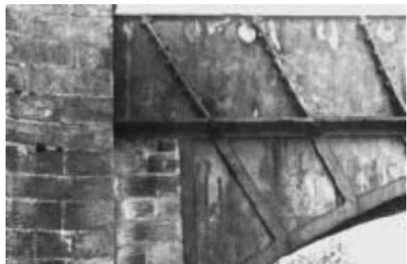
Fig. 21: Pont Cysyllte Viaduct, 1805. (Sealey)
