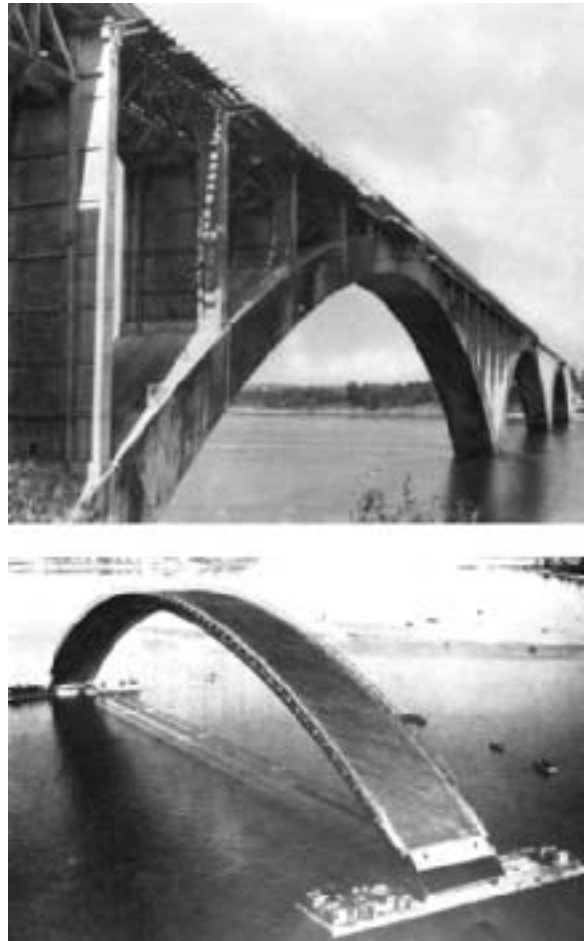
Fig. 17: (a) Elorn Bridge with three spans of 186.4 m each, Freyssinet, 1930. (b) Self-supporting centering used to construct the Elorn Bridge being floated into place. (Wittfoht)
