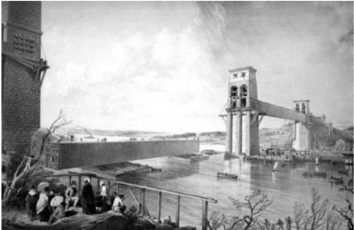
Fig. 70: A tube being moved into place on the Menāi. (Walker)
