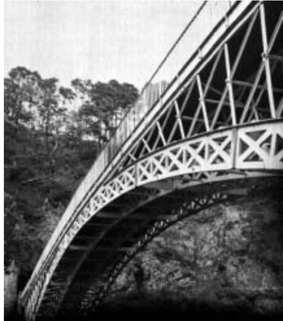
Fig. 19: Craigellachie Bride, cast-iron arch. Telford, 1810. (Ruddock)
