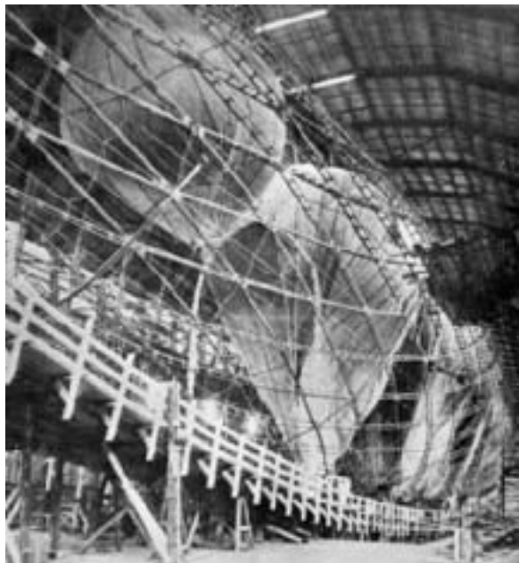
Fig. 60: Plywood airframe of SL-1, under construction. (Meyer 2 )
