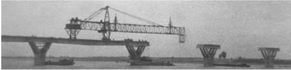
Fig. 41: Kosi Bridge near Kursela, India, 1000 m long bridge built with 50 m long pre-cast girders and piers with “platforms” 15 m long to extend distance between piers. (Wittfoht)
