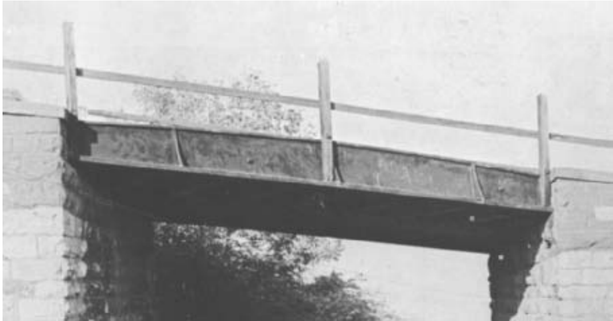
Fig. 32: Typical cast-iron girder bridge for railroads in England, early 19 th century. (Sealy)
