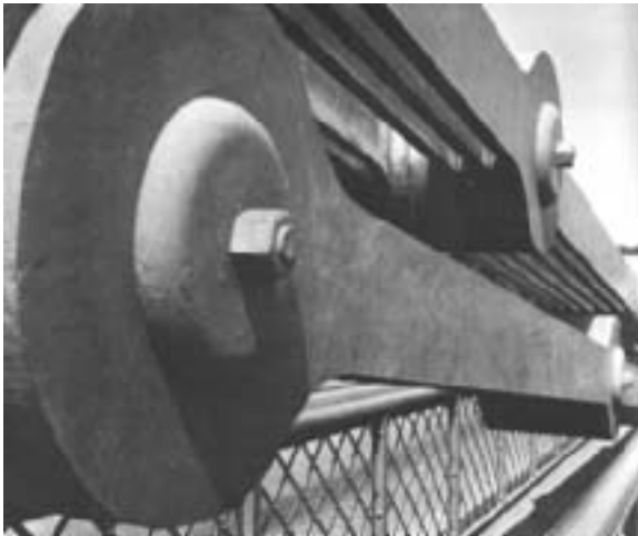
Fig. 30: Menai chain link (replacement, similar to original). (Ellis)
