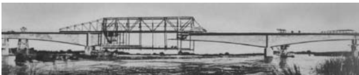
Fig. 51: Railroad bridge across the Lualaba River at Kongola in the former Belgian Congo, first reinforced concrete bridge built using a launching gantry, 1938. (Wittfoht)
