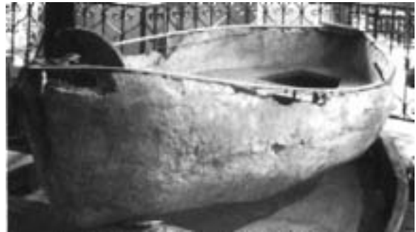
Fig. 4: Ferro-cement boat, Lambot, 1848. (Prade)
