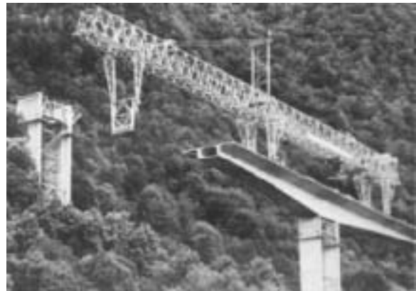
Fig. 61: Chillon Viaduct, Montreux, Switzerland. Construction view. 1970. (Wittfoht)
