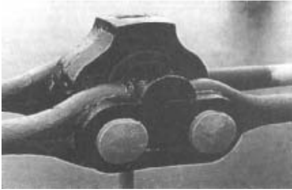
Fig. 29: Chain link and hanger connection of Union Bridge. (Sutherland)
