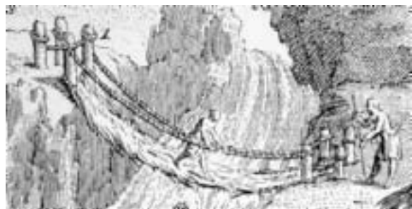
Fig. 3: Basic three-rope suspension bridge. (Brown)
