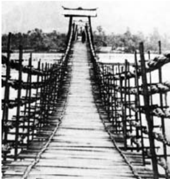
Fig. 4: Quan-Xian Bridge, with bamboo suspension cables. (Peters 2 , after Tang)
