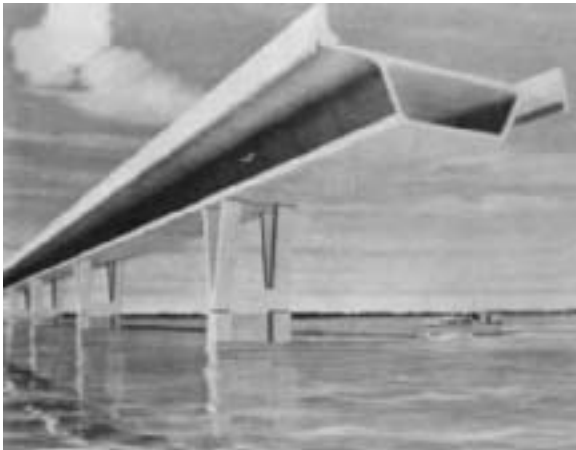
Fig. 67: General view of Long Key Bridge, Florida, USA. 3.7 km total length with 36 m spans. Muller and Figg, 1976. (Podolny and Muller)
