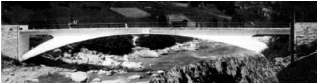
Fig. 37: Tavansa Bridge, 1905. Maillart's improved box section design with material removed from areas of spandrels where cracking was observed in the Zuoz and Bilwil bridges. (Billington 1 )
