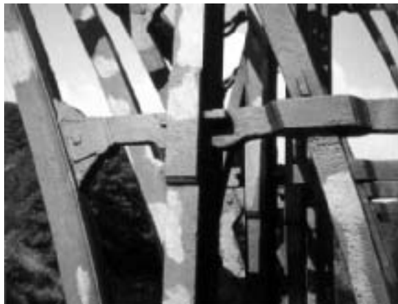
Fig. 43: Detail of Ironbridge showing timber-like connection. (Brown)
