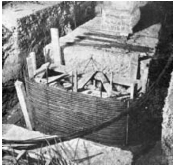
Fig. 19: Prestressing system used by Freyssinet to jack the tendons of the tie beams in the Gare Transatlantique at Le Havre, 1934. (Freyssinet)
