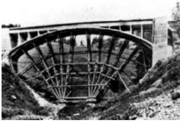
Fig. 8: Flienglibach Bridge, first deck stiffened arch built by Robert Maillart, 1923. (Billington 1 )
