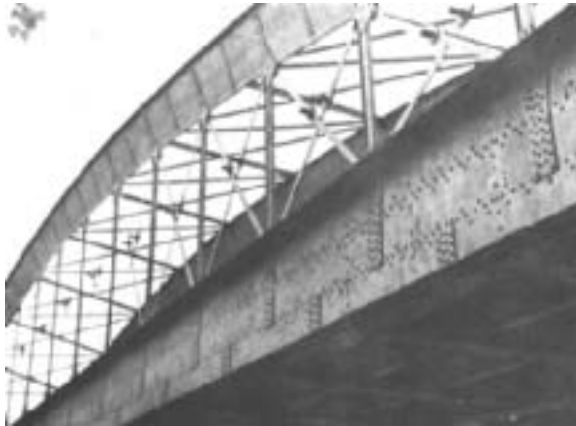
Fig. 74: Windsor Bridge, tied-arch, compression tube with triangular section, I.K. Brunel, 1849. (Sealy)
