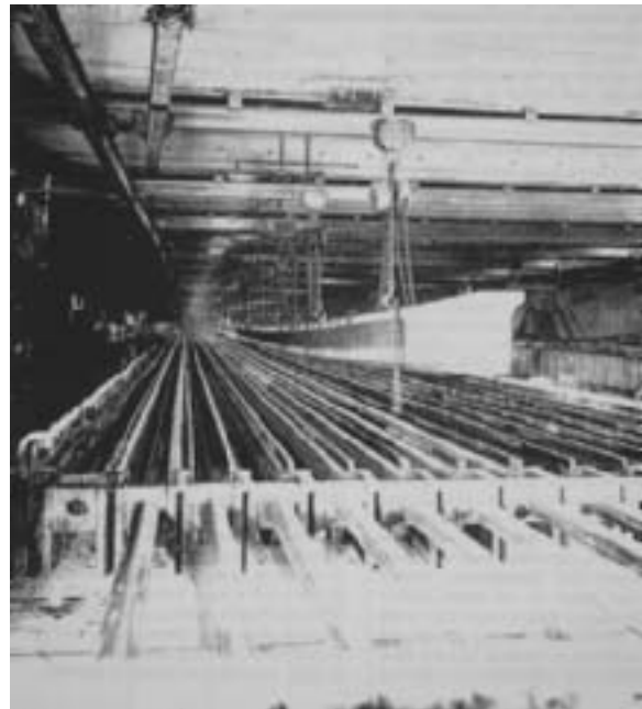
Fig. 26: Production line for Ewald Hoyer's divisible prestressed concrete girders precast in 100 m lengths. (Grote and Marrey)
