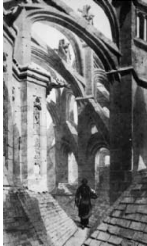
Fig. 12: Flying Buttress. (Recht)
