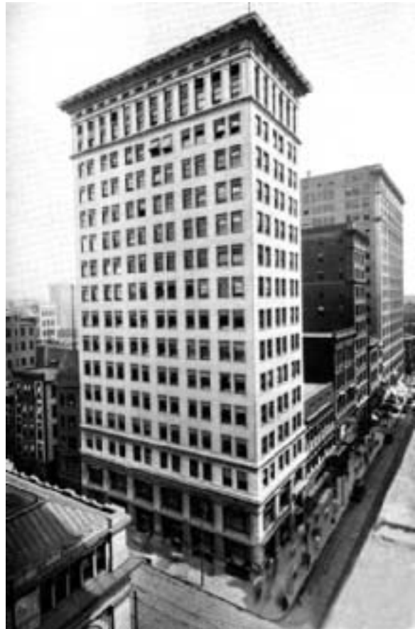
Fig. 16: Ingalls Building, 16 story reinforced concrete structure designed and built by the Ferro-Concrete Company, Cincinnati, 1902. (Collins)
