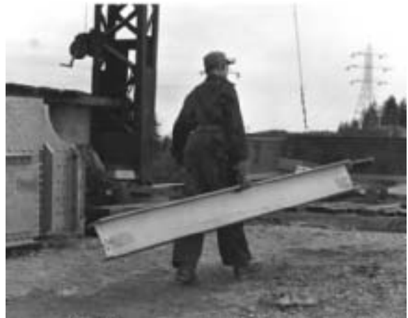
Fig. 36: The Arvida Bridge, Quebec. All-aluminum arch, span = 91.5m. 1950. (Dominion Bridge)
