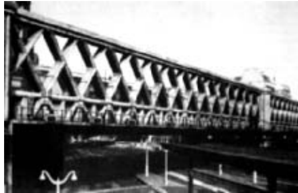
Fig. 10: Trussed reinforced-concrete bridge, the Rue Lafayette Bridge over the railway lines at the Paris-East Railway Station with a span of 71.87 m and a depth of 10.40 m, Caquot, 1928. (Deinhard)
