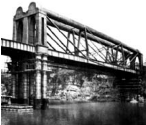
Fig. 75: Chepstow Bridge, suspension system stiffened and strutted by compression tube with circular section, I.K. Brunel, 1852. (Sealy)
