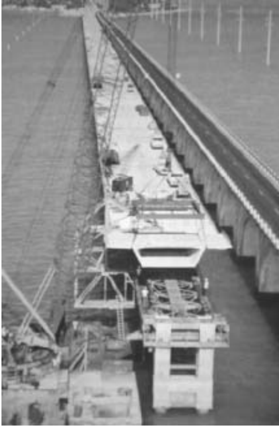
Fig. 59: Long Key Bridge, Florida, USA, construction view. 3.7 km total length with 36 m spans, Muller and Figg, 1976. (AFPC et al.)
