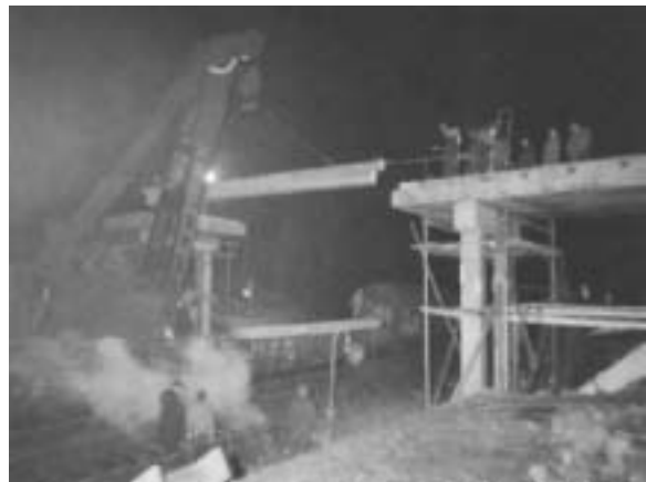
Fig. 40: Erection of precast prestressed concrete girders over railway tracks in Germany to construct a field access bridge. (Wittfoht)
