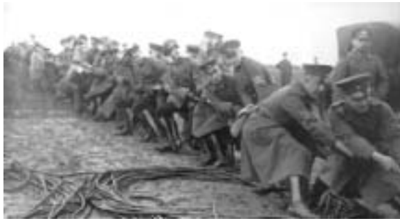
Fig. 10: View of ground handling procedure requiring many men. (Knäusel)
