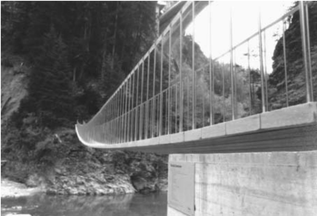
Fig. 26: Stressed ribbon bridge using stone and stainless steel prestressing bands. Suransuns Bridge, Graubünden, Switzerland. Jürg Conzett, 1999. (Dooley)
