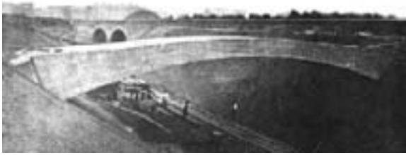
Fig. 4: One of the first recorded concrete bridges, Fowler, 1869, England. (The Railway Gazette)
