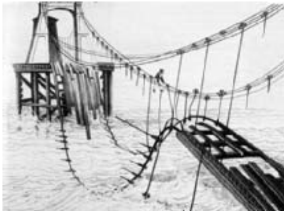
Fig. 2: Brighton Chain Pier, Samuel Brown, 1823. Damage caused by wind-induced oscillations in 1833. (Peters 3 )
