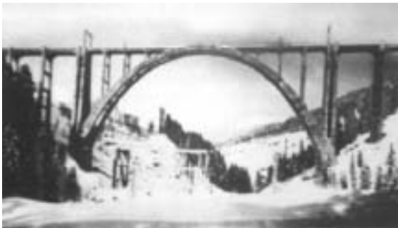
Fig. 5: Langwies Viaduct, reinforced concrete arch with 100 m span, Züblin, 1916. (Wittfoht)
