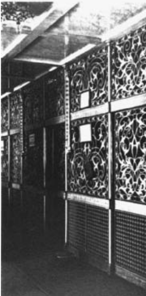
Fig. 31: Aluminum staircase and elevator enclosure, Monadnock Building, Chicago, 1892. (Nichols)
