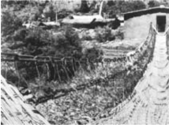
Fig. 6: Docsum Sempa Bridge, with iron-link chain-cables. (Peters 2 , after von Schulthess)
