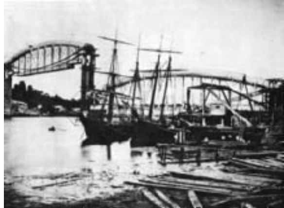
Fig. 76: Saltash Bridge, lenticular truss, compression tube with elliptical section, I.K. Brunel, 1859. (Sealy)
