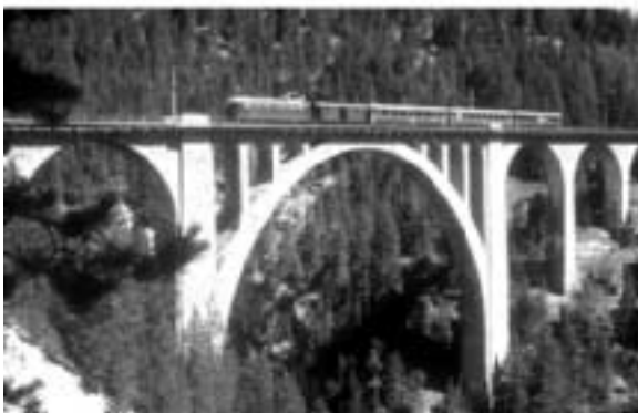
Fig. 23: Stone viaducts built at the turn of the twentieth century. Langwasser Viaduct (1902) and the Wiesener Viaduct (1908). These are among the slenderest constructions of their type. Both are located in Graubünden, Switzerland.
