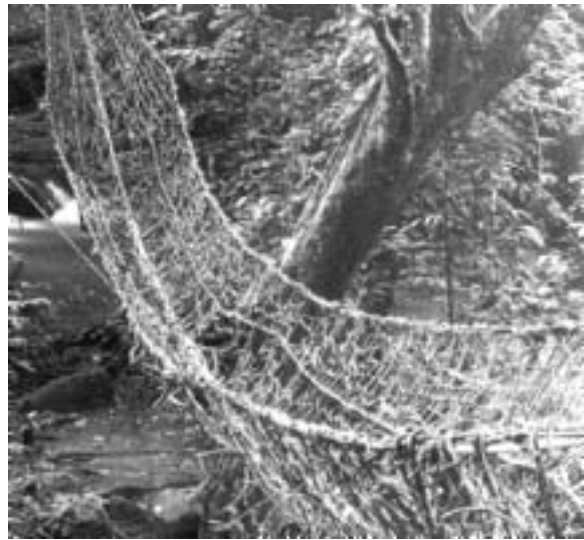
Fig. 1: Three-cable suspension bridge manufactured using vines. (Brown)
