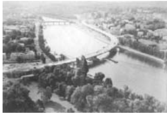
Fig. 60: Saint Cloud Bridge, on Paris Ring Road over the Seine River, France, 1975. General view showing difficult geometry and the use of three-dimensional pre-stressing to counter torsion. (Podolny and Muller)
