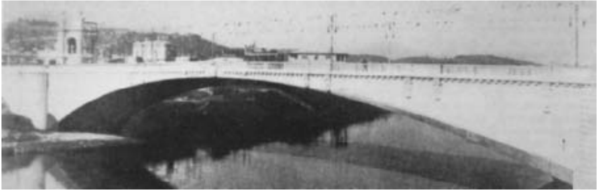
Fig. 7: Risorgimento Bridge over the Tiber River in Rome, first deck stiffened arch, Società Porcheddu, 1911. (Hennebique Archiv)
