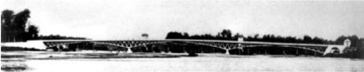
Fig. 16: Bridge at Le Veudre, France, 3-hinged arch with triangulated spandrels with three spans of 72.5 m each, Freyssinet, 1907. (Wittfoht)
