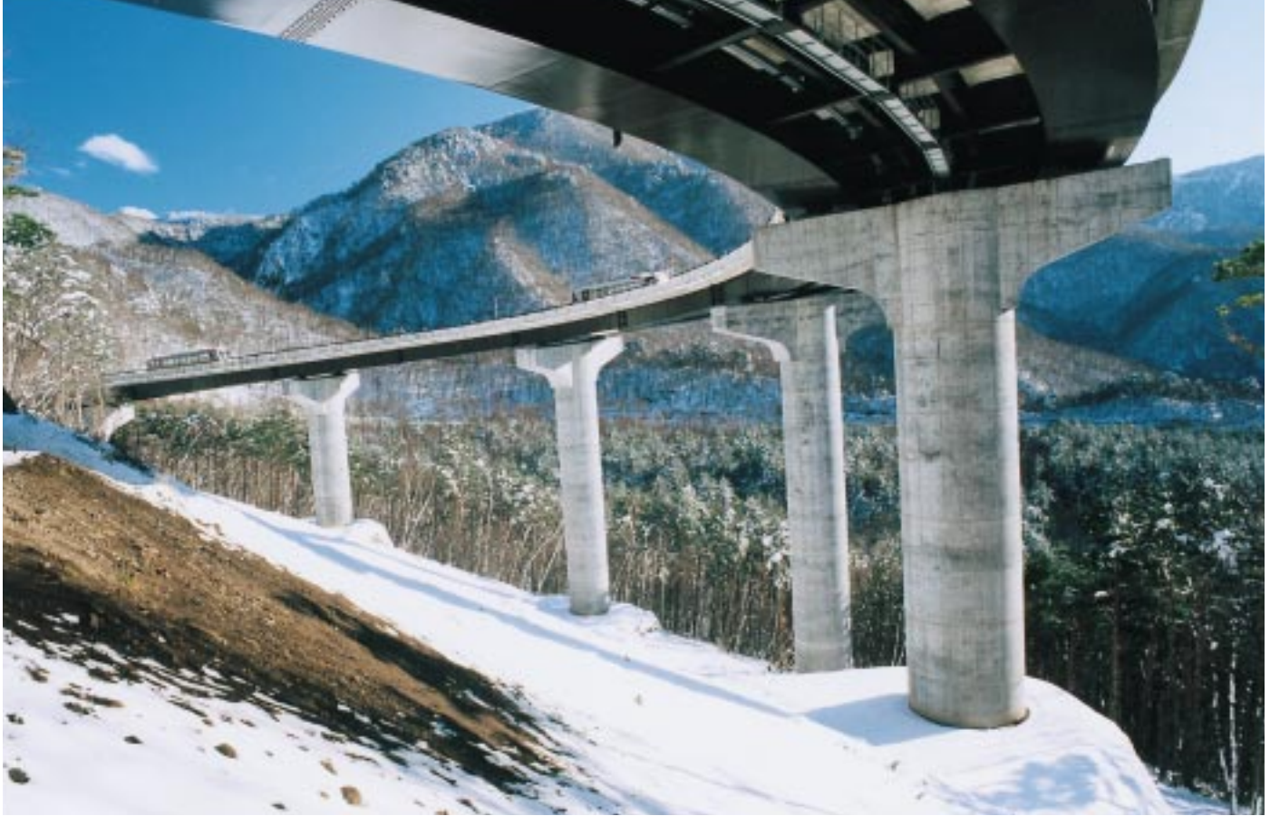
Bridges such as this eliminated the need for a succession of hairpin turns on the Shiga Route.
