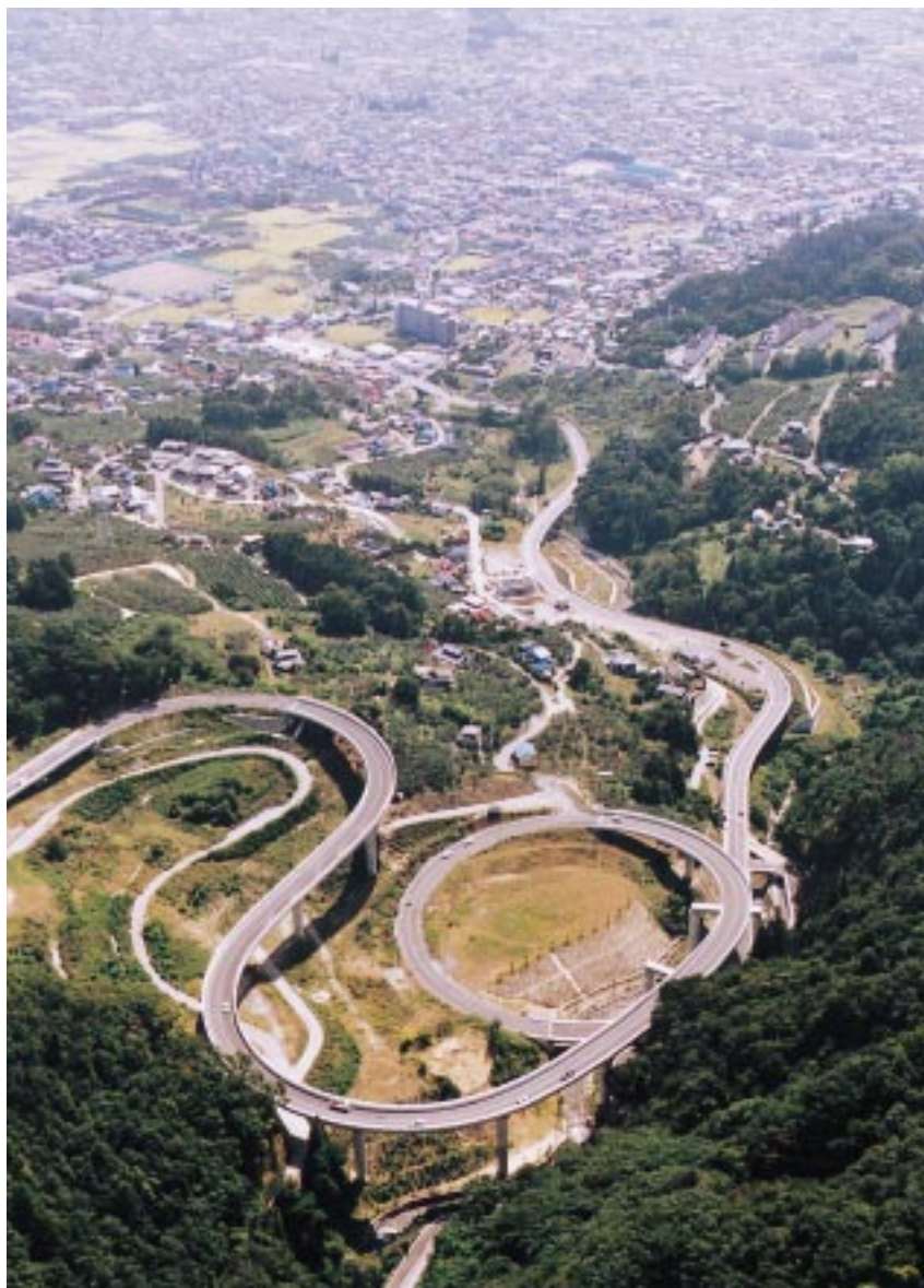
The spectacular Shinkoji loop bridge facilitated access to Iizuna Kogen.
