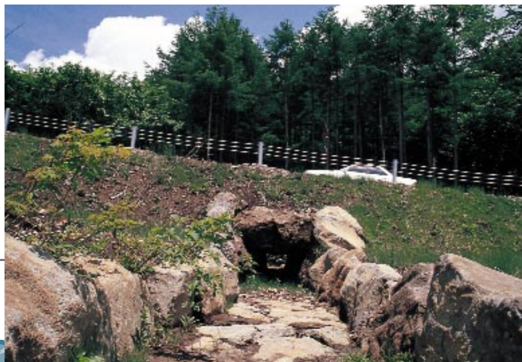
In Shiga Kogen, tunnels constructed under roads allow woodland animals to cross safely.
