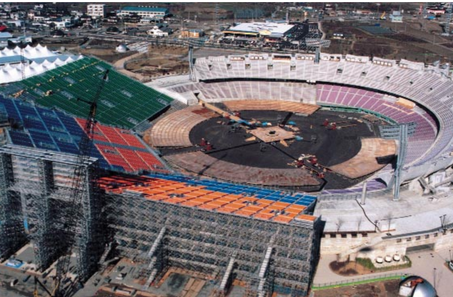
Temporary spectator stands at the stadium for Opening and Closing Ceremonies.
