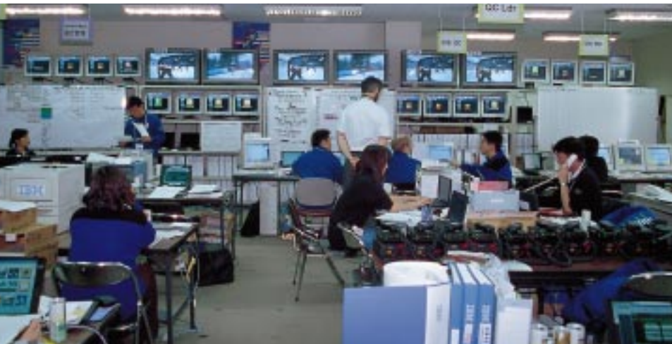
During the Games, all systems were monitored at the Systems Operations Centre (SOC).
