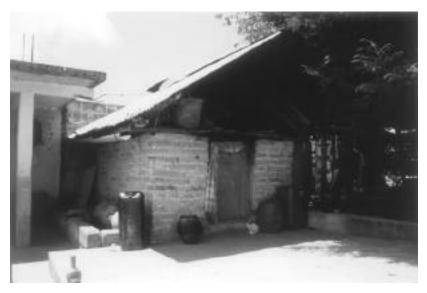
**Figure 6.** Modern brick-and-cement steambath with corrugated tin rain shelter, Oxchuc center (© 1997 by K. P. Groark).
