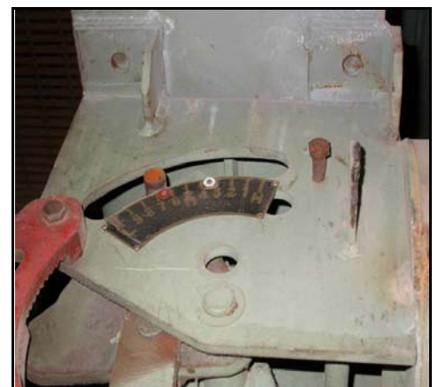
Figure 3. An exemplar constant support hanger scale.
