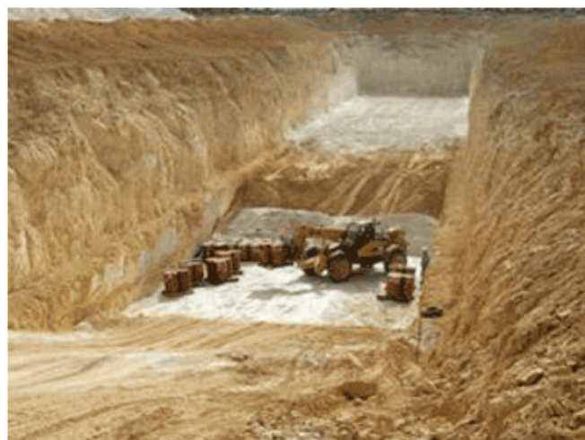
Above, Australia's only low level waste repository at Mount Walton, Western Australia. It is only for WA waste. Note the drums of radioactive waste sitting in the middle. When the trench is full, the contents are then buried under topsoil and various other layers to prevent wind and rain reaching them. The aim is never to dig the contents up once the trench is closed.
