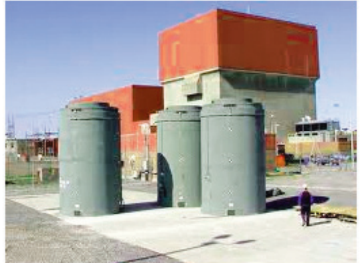
Typical dry cask storage of spent nuclear fuel. The casks to be sent to Australia will be smaller but there will be many more than pictured here.
