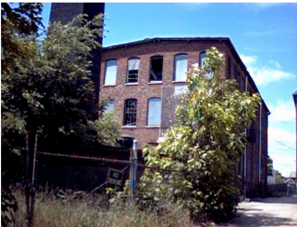
Figure 1: Photo of old mill building at 1 Mashapaug Street from south side
