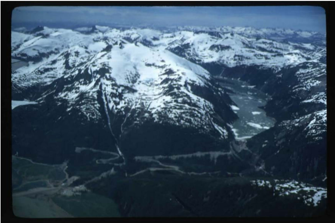
The hydroelectric development at Snettisham, south of Juneau, drawing water from an alpine lake.
