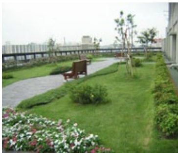
"A green roof on BROTHER INDUSTRIES, LTD." Mizuho Ward, Nagoya City, Japan
