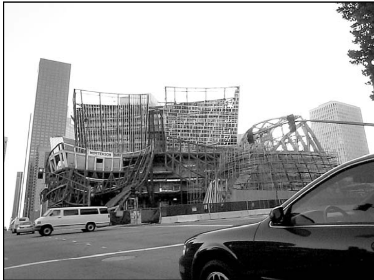
Disney Center under construction, Los Angeles. March 2002 [Photo by Torin Monahan]
