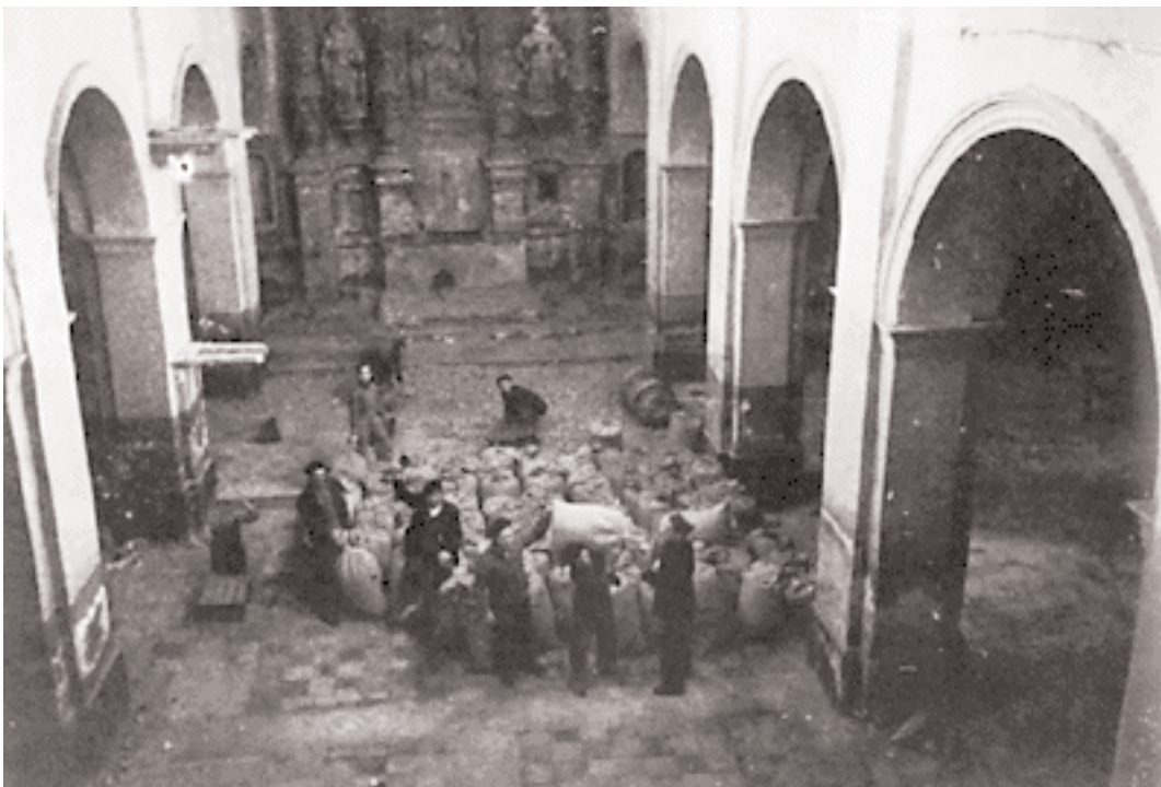
a church is used to store agricultural produce
