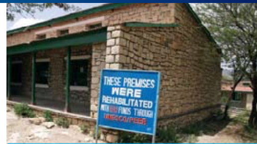
A section of the buildings at Amoud University (Somaliland), rehabilitated by UNESCO PEER
