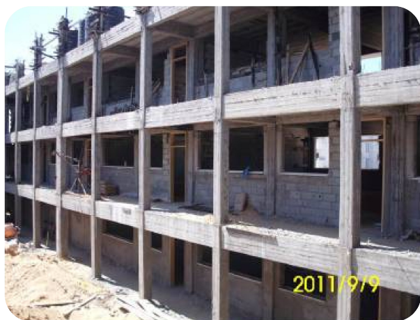
Construction of School in Tel Alwah by UNRWA
