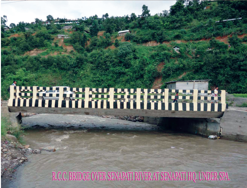
MARAM TO PURUL ROAD UNDER SPA.
