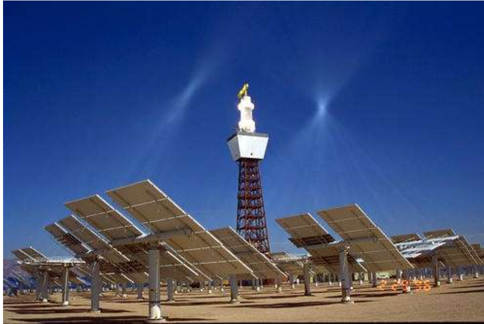
Figure 6-22 Picture of Central Receiver Plant
