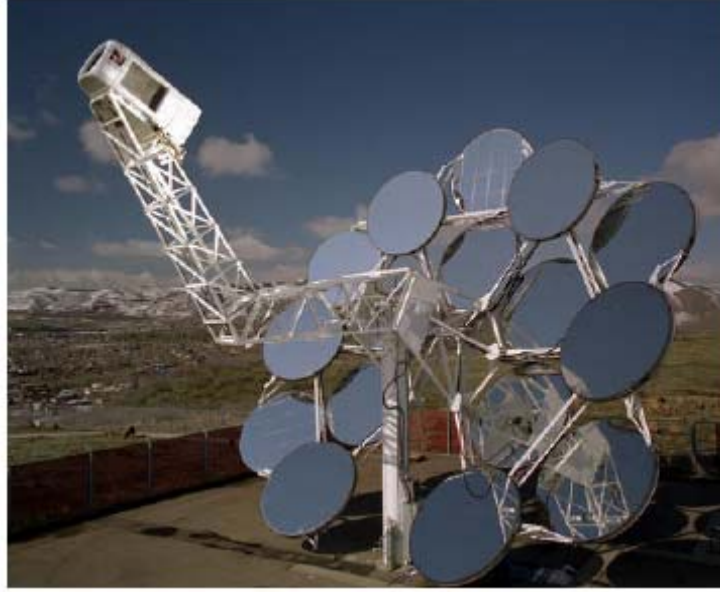
Figure 6-27 25-kW SAIC Dish/Engine System at the DOE Mesa Top Thermal Test Facility
