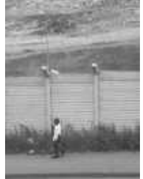
The fence separating the dumpsite from the surrounding communities.
