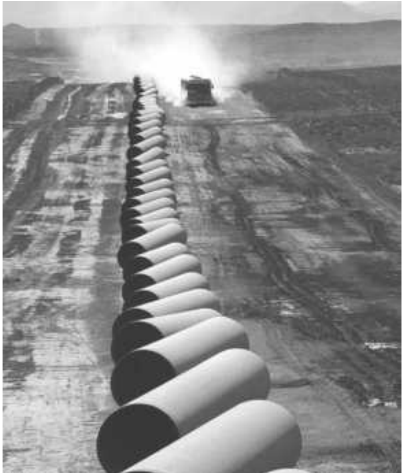
Segments of the Baku-Ceyhan pipeline await assembly.
