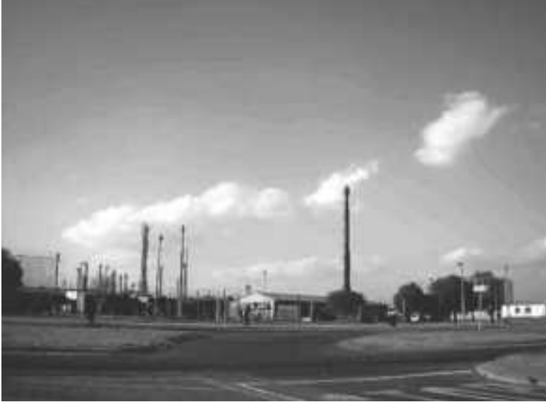
Sasol gas flaring. Such flaring is alleged by environmentalists to be in breach of South African law.
