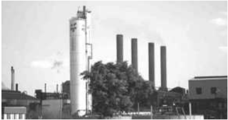
Sasol's Sasolburg plant, seen from the south.
