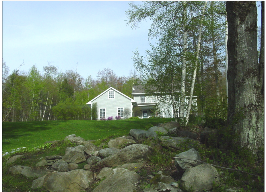
Figure 5- Recent construction along Notch Road in Bolton
