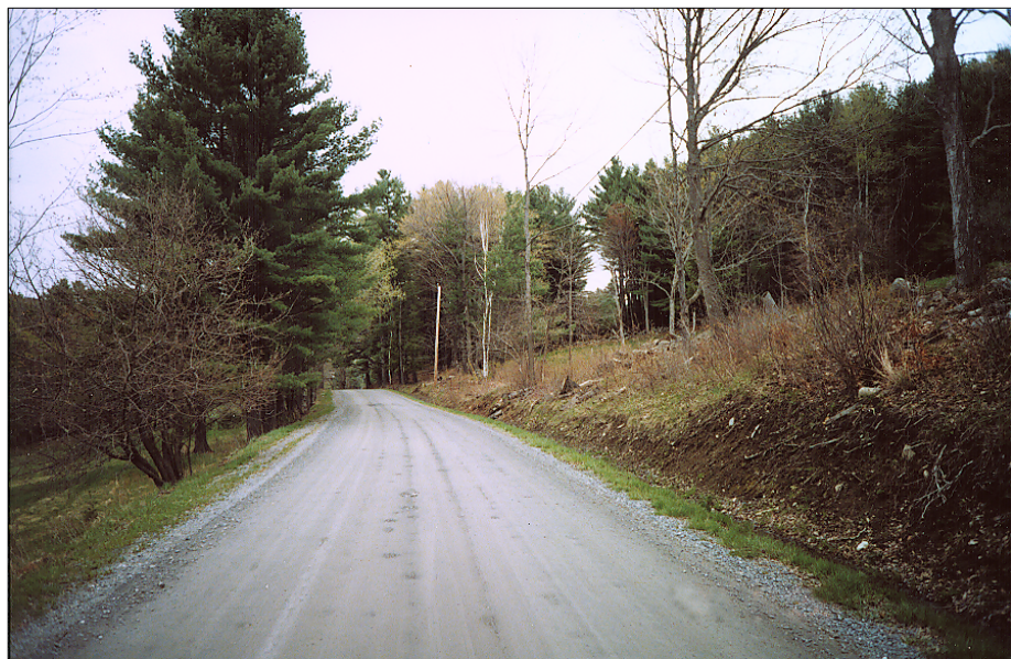
Figure 4- Cleared roadside with preserved pine
