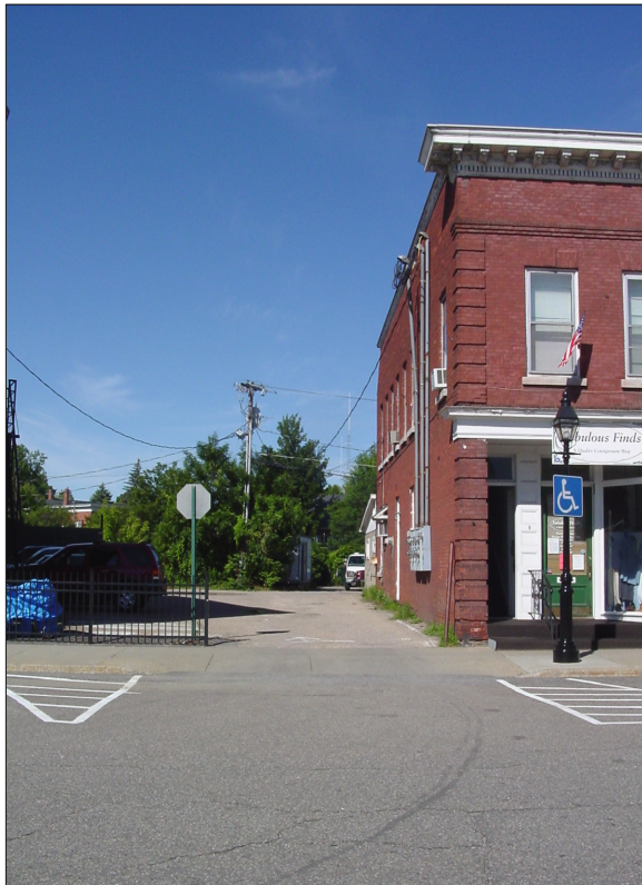
Figure 11- Urban overhead lines placed in the “back alley” in the Village of Essex Junction
