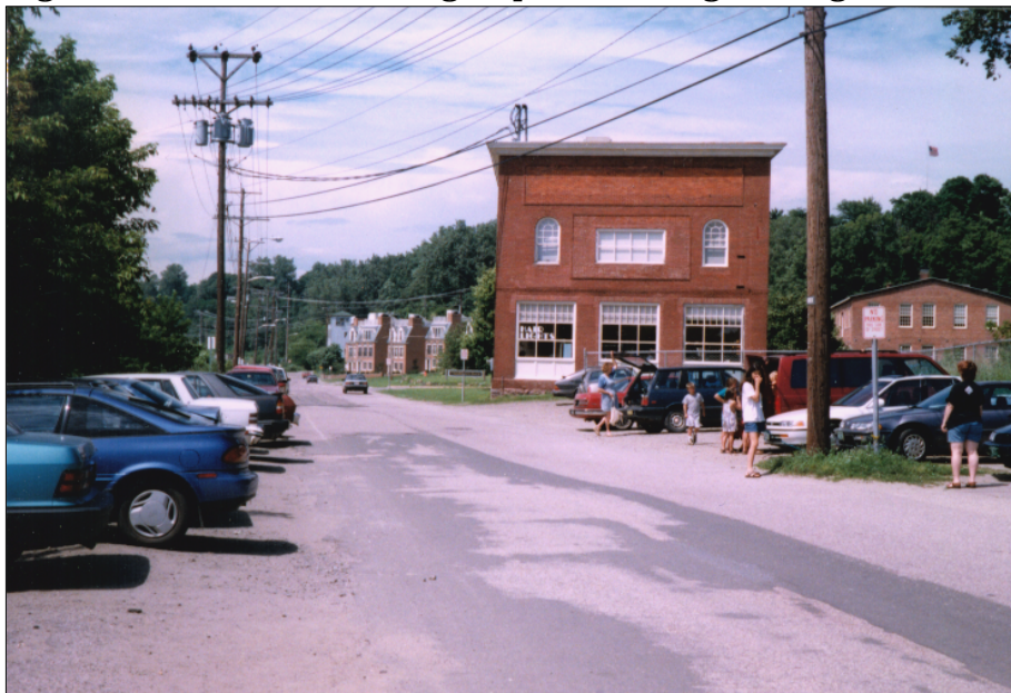
Figure 10- Lake Street in Burlington prior to undergrounding.
