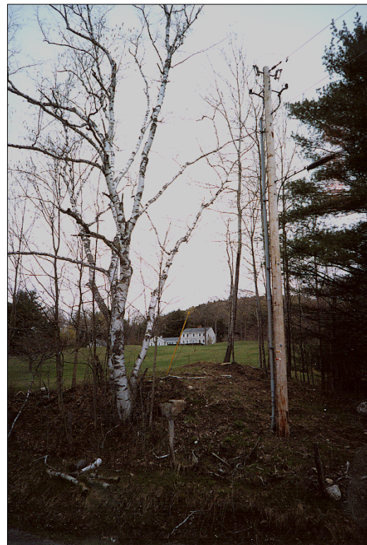
Figure 3- Blood Brook Road showing riser pole
