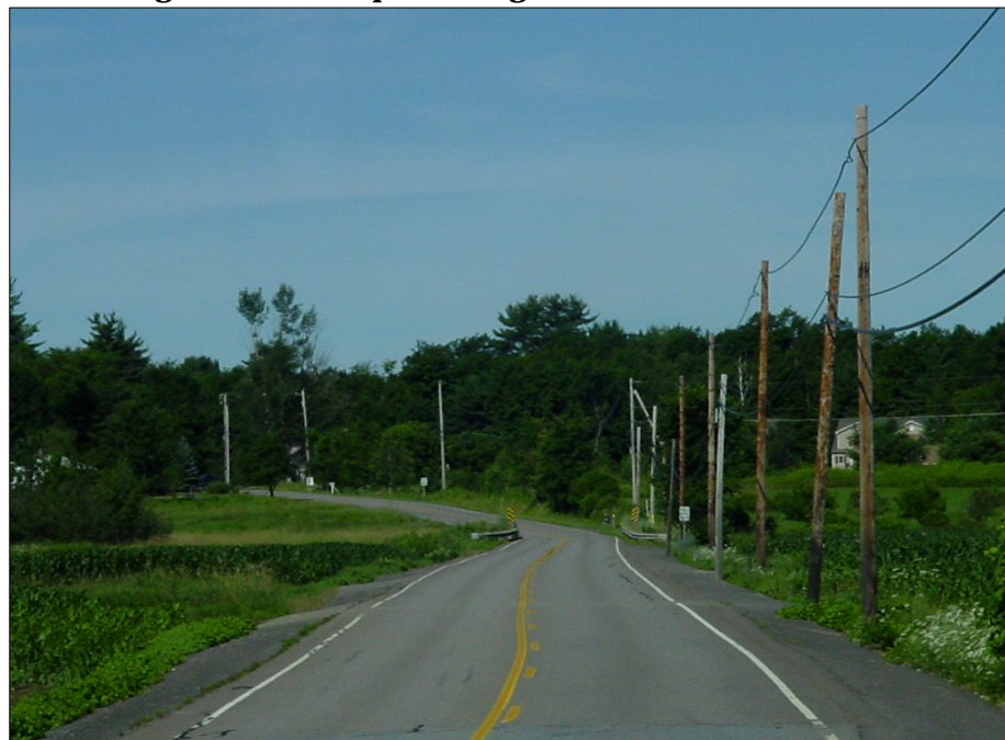
Figure 9- “Dead” poles along road – loss of order and intactness.
