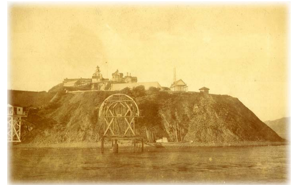
Construction of an early visual Tide Elevation Recorder at Alcatraz Island
