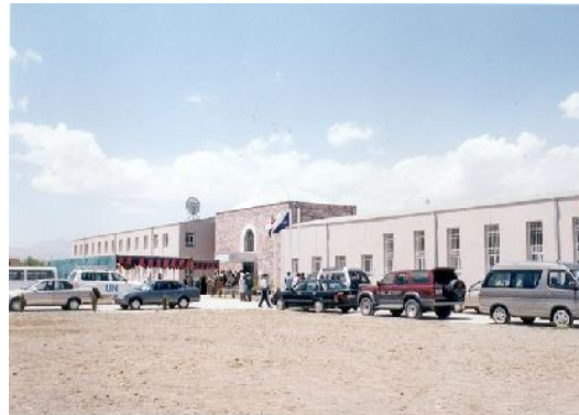
Anti-Tuberculosis Center in Kabul constructed by Japan
