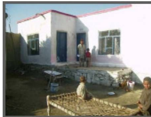
Shelters for returnees in Nangarhar (Photo provided by FAO)
