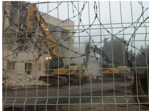
Demolition of Shepherd's Hotel, January 9, 2011
