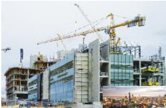
Fiona Stanley Hospital: Massive and complex, on schedule.
