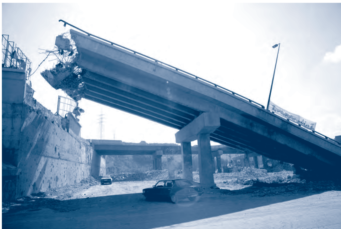
Photo © Simon Conway - Destroyed bridge on the road from Beirut to Tyre, Lebanon, September 2006
