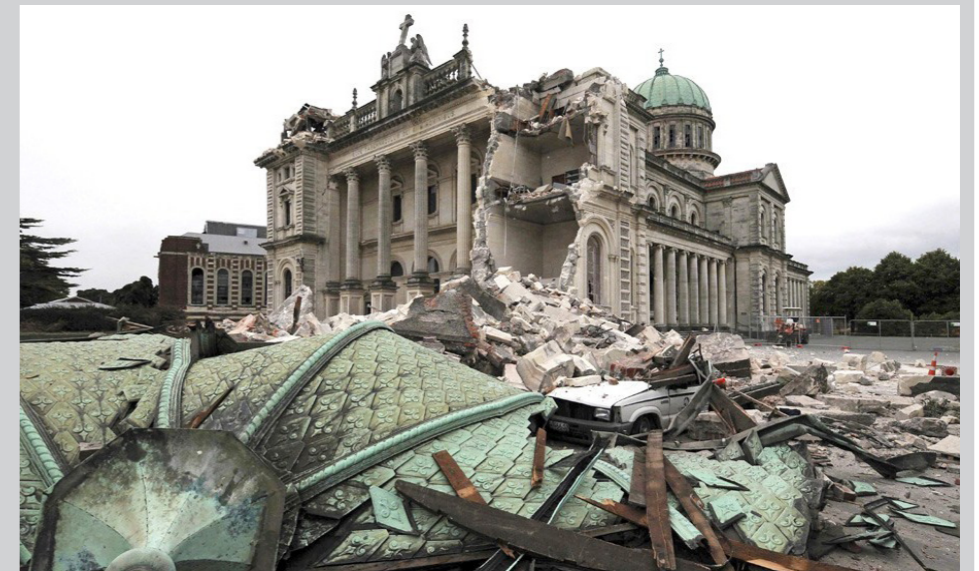
Another quake hits Christchurch, this time more devastating. Many buildings like this Cathedral were brought down.
