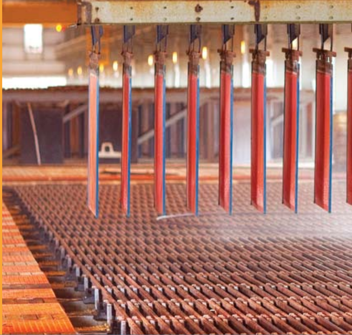
Tenke Fungurume Mining Processing Plant, Democratic Republic of Congo
