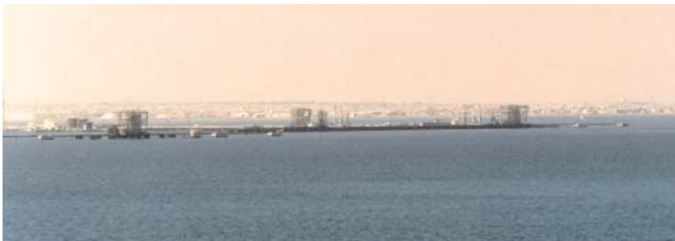
Sitrah Oil Terminal—No. 1 Island Wharf (left) and No. 2 Wharf (right)
