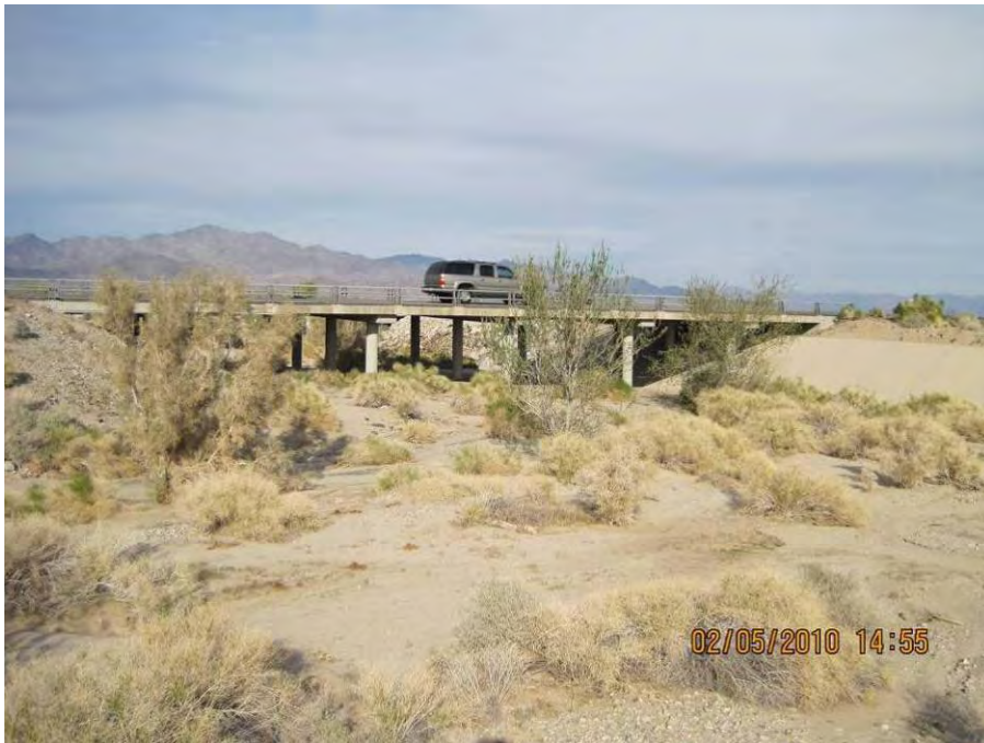
Figure 20. Interceptor channel passes under I10 (flow away from viewer)
