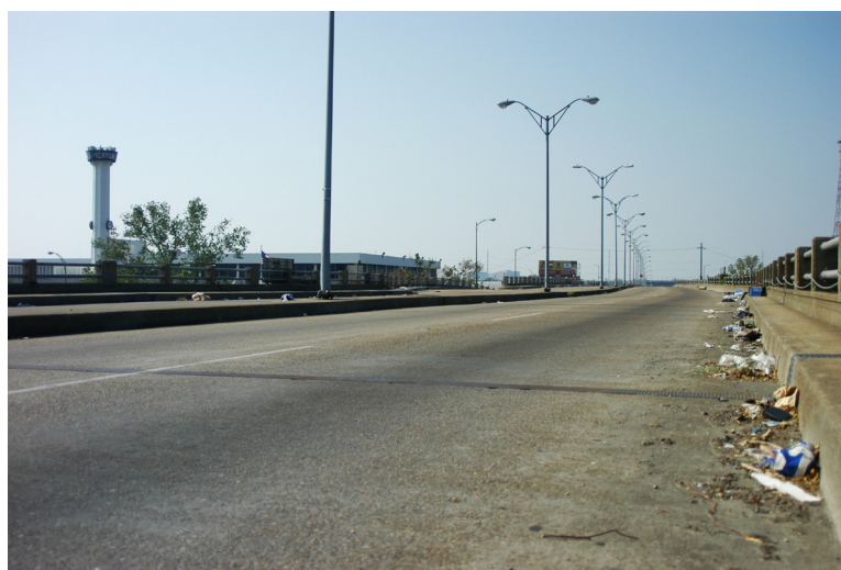
ABOVE: Broad Street bridge, where thousands of prisoners were left for days.
