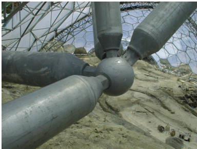
Fig. 10 The bottom chord node
