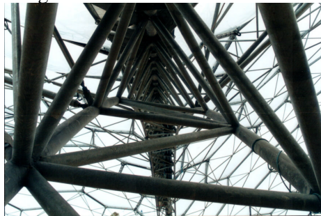
Fig. 11 View of the arch
