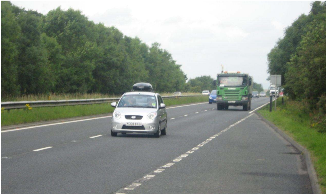
Figure 6: The A1 between Alnwick and Morpeth.
