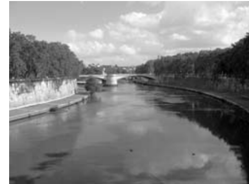
Above: Stretch of the Tiber River above the Ponte Garibaldi showing the resultant sectional displacement of the city from its river. The embankment walls did much more than just protect the city from flooding—they severed the city from the river. This infrastructural solution essentially depressed the river below the level of the city.
