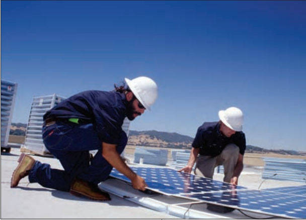
Installing PV system.
