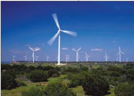
Trent Mesa Wind Power Facility (150 MW), Sweetwater, Texas.
