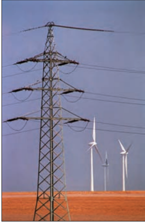
Wind farm with transmission tower.
