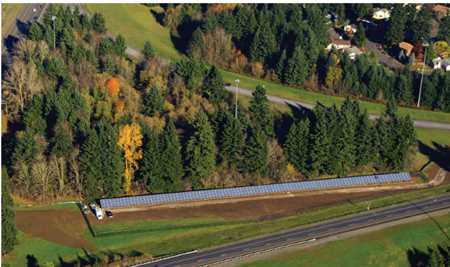
This aerial view of the Oregon Solar Highway shows the PV Powered inverter located at the west end (left side) of the long array of solar modules.
