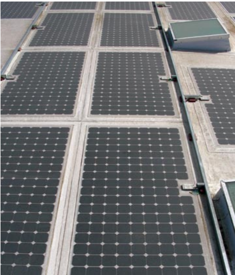
Photovoltaic solar panels are integral to the single-ply membrane roof
