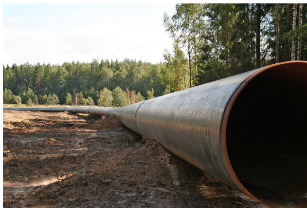
Pipeline construction in Alberta forest
