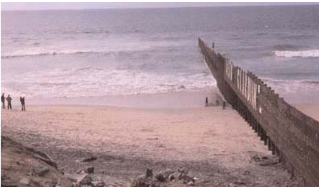
seawall forming part of the US-Mexico border
