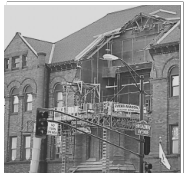
Courthouse construction has begun... Whoopie!!
