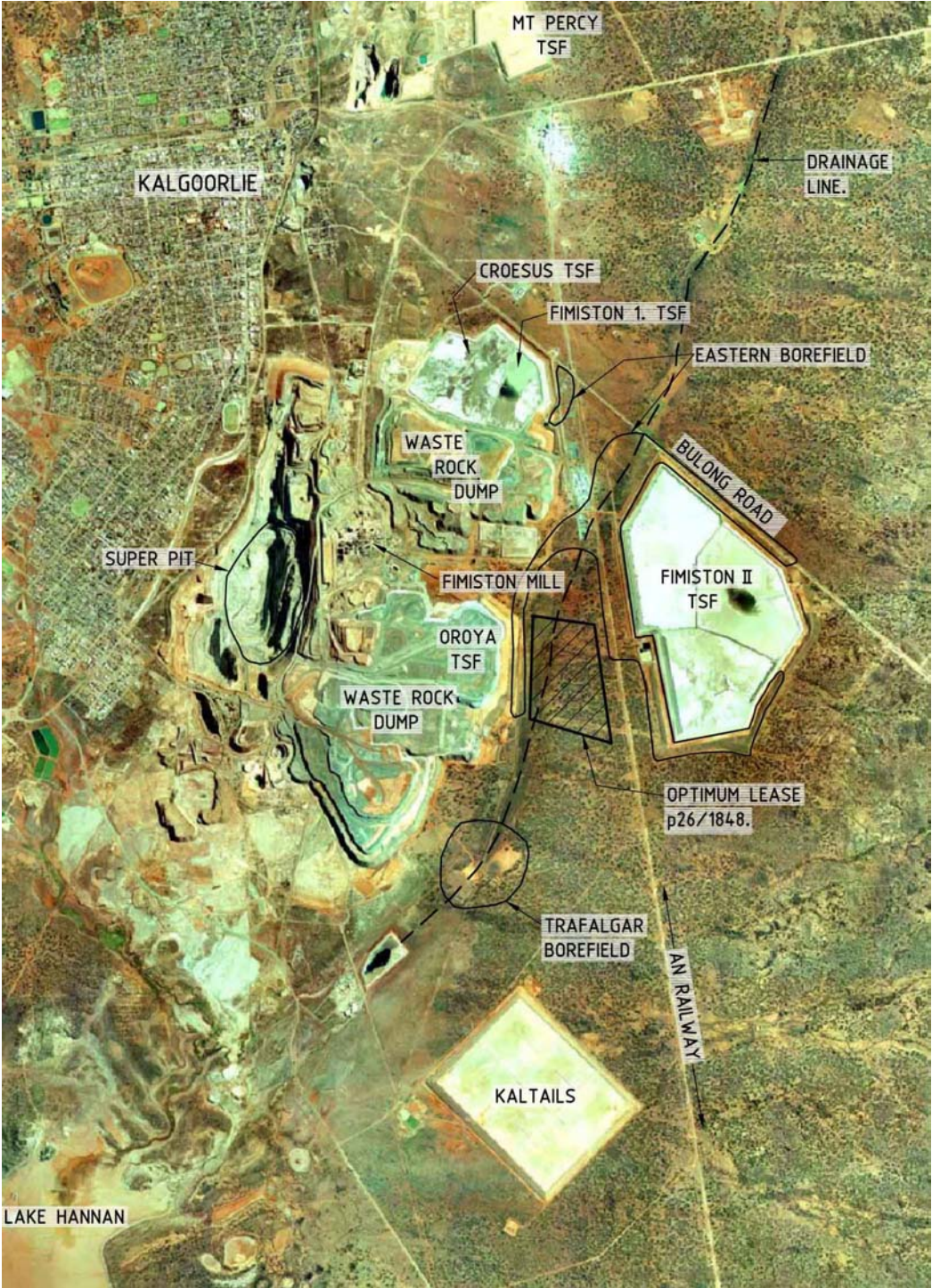
Figure 1 Aerial Photograph of the Site Showing Main Features
