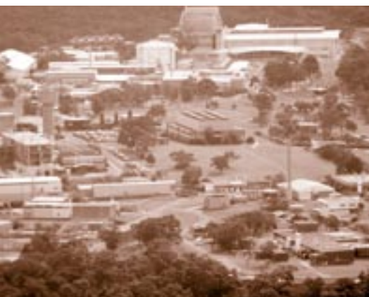
Aerial view of Lucas Heights. Silex building 64 – bottom right.
