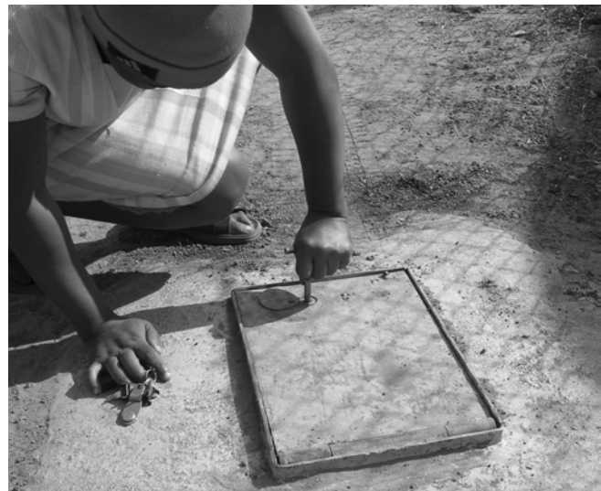
A Phiri resident opens a prepaid meter box that has been set in concrete since the pilot project in Orange Farm showed that meters above the surface were too easily broken.
